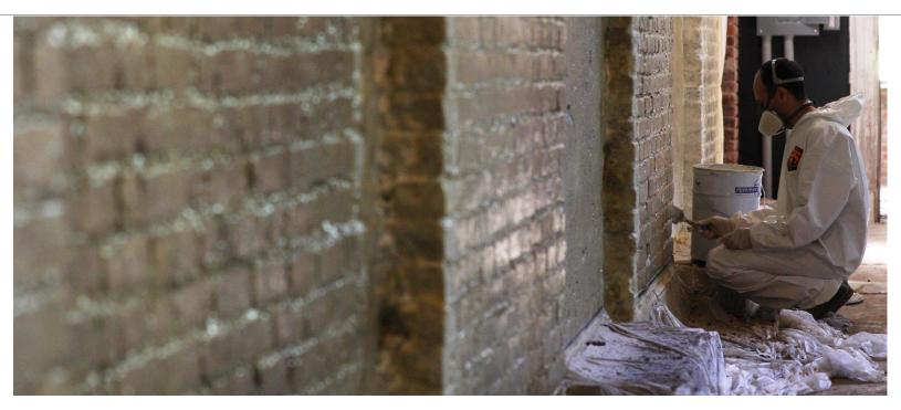
Rebirth in progress. Latex being applied to the natatorium's brick walls. (Courtesy Studio Otero-Pailos)
